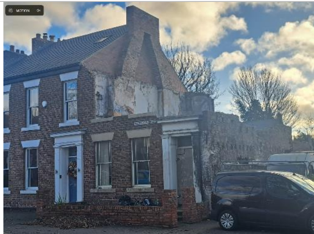
Photograph 1: Building overview from south looking north (front elevation) .
